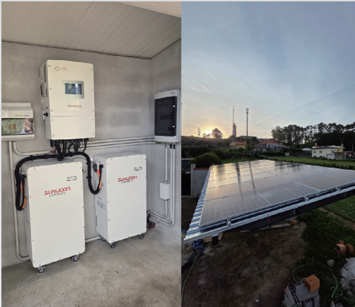
Atrix Max + 12kW/32kWh RESS Atrix Max + system RESS for Residential Building
