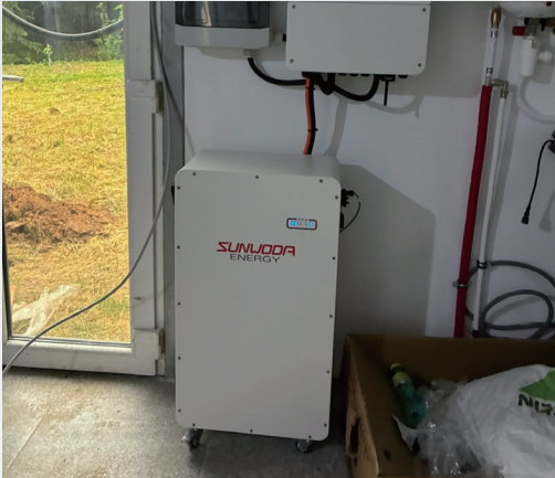
Atrix Max + 6kW/16kWh RESS Atrix Max + system RESS for Residential Building
