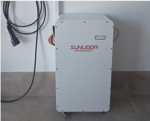
Atrix Max + 16kWh RESS Atrix Max + system RESS for Residential Building
